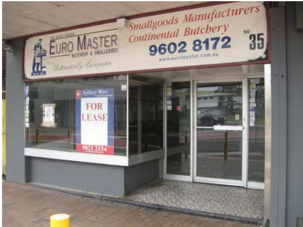
Figure 18 — detail of a typical shop front at 29–33 Scott Street with 1960s floor tiles and c1970s aluminium-framed fenestration.
