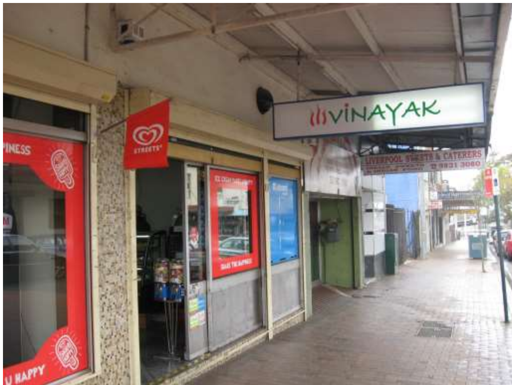
Figure 15 — the under-awning view of the shop fronts of the Imperial Buildings. The wrought steel trusses, with timber purlins in between, was typical of the inter-war period. NBRSPartners, September 2015.
