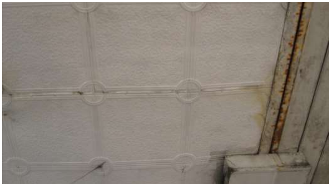
Figure 19 — pressed metal ceiling under the awning of 29–33 Scott Street is 1930s–50s. This Wunderlich pattern is still fairly common across Sydney.
