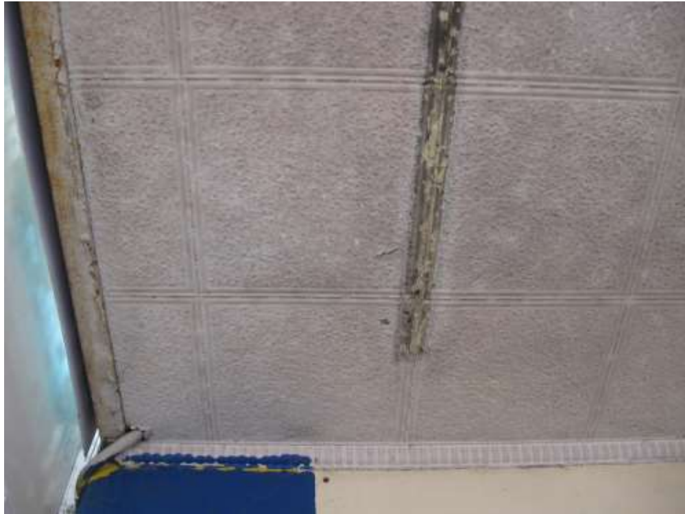
Figure 22 — the soffit and cornice of the awning at 37A Scott Street have a Wunderlich pattern that was sold in the 1950s. NBRSPartners, September 2015.
